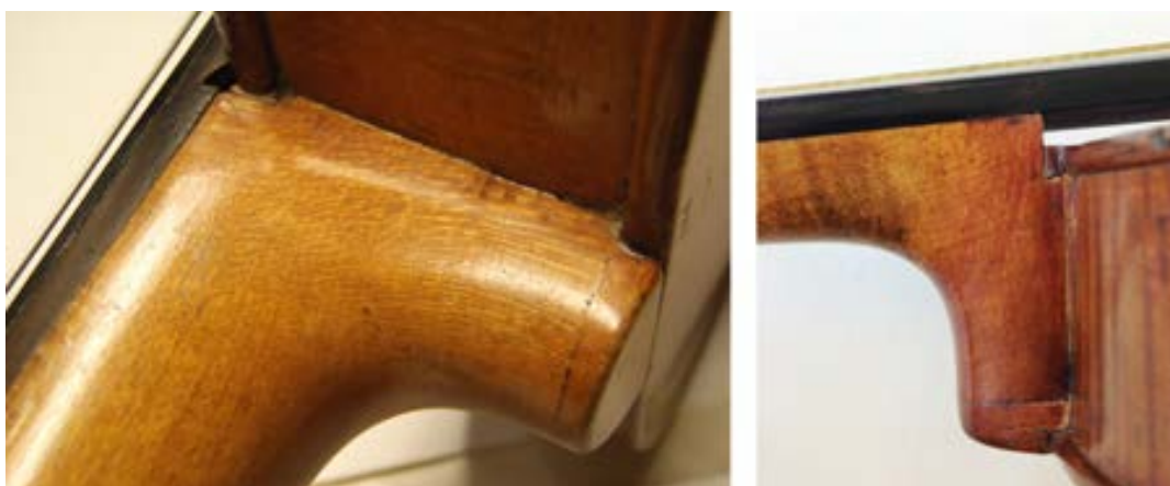
Figure 4.52. Detail of neck heel of two violins by Boussu. Left to right: (a) neck heel of a violin dated 1750 (MIM inv. no. 2781; database code BJB5001vn), (b) modified neck heel of a violin dated 1751 (MIM inv. no. 2785; database code BJB5101vn).
