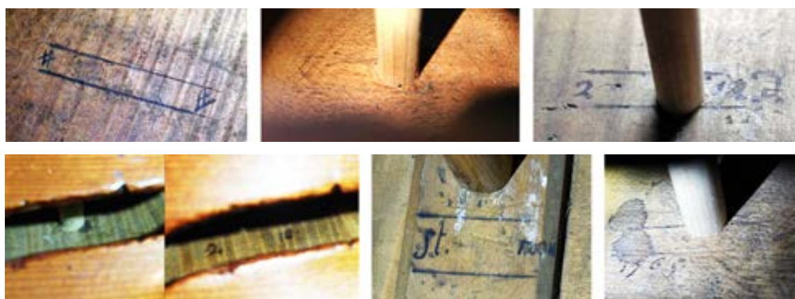
Figure 4.12. Six examples of soundpost position markings. Top row, left to right: (a) soundpost marking in a cello from 1757 (MIM inv. no. 1372; database code BJB5701vc), (b) soundpost marking in a violin from 1758 (database code BJB5801vn), (c) soundpost marking in a viola from 1759 (database code BJB5901va). Bottom row, left to right: (d) soundpost marking in a violin from 1759 (database code BJB5903vn), (e) soundpost marking in a double bass from 1760 (MIM inv. no. 2014.324; database code BJB6002db), (f) soundpost marking in a violin from 1765 (database code BJB6501vn).
